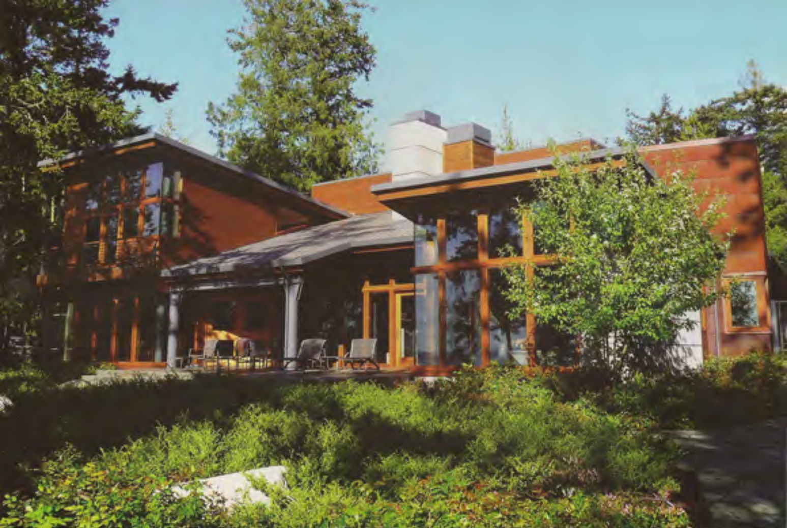
Located just outside Roche Harbor, this contemporary Northwest home uses a combination of materials including metal weathered clad siding, Western Red Cedar and architectural grade concrete. Demetriou Architects
