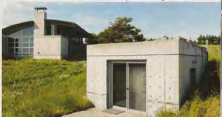
Near wind-swept Eagle Cove on the South end of San Juan Island, this modern custom home sits quiet and peaceful, the detached "bunker" features two beds, shower and large skylight. Suyama Peterson Deguchi Architects
