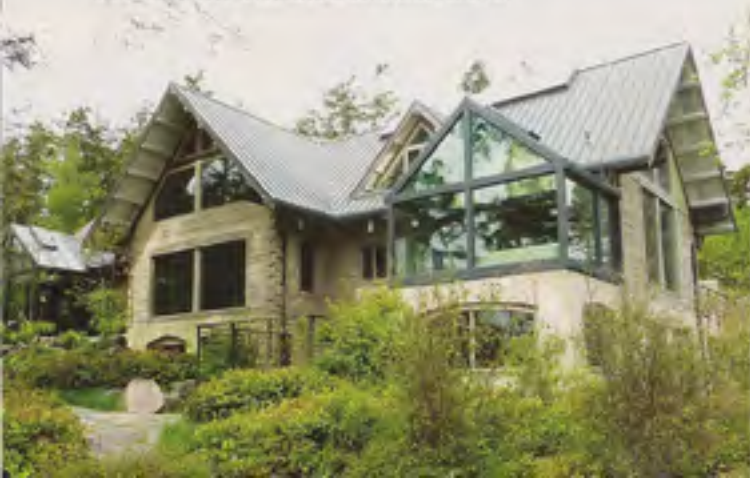
This home utilized the original solid timber walls. Lowe Construction then constructed a new roof line and extensive use of steel and glass rooms to create and maximize it's view, complete with an indoor pool. 4d Architects w/ David Kinderfather AIA
