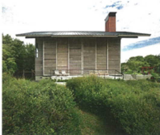
The massive exterior shutters, 20 feet tall, close up the home, controlling light and solar-heat gain. The grounds were designed by Steve Schramm of Island Gardens. The home was built by Dan Lowe of Lowe Construction in Friday Harbor.
